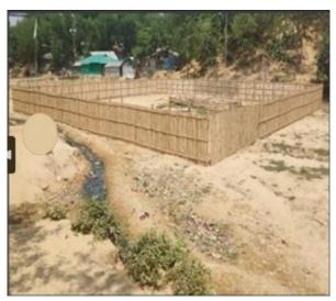
This construction of this plant consists of site preparation, tank platform construction, Different tanks / solar system / Felxigester / Drying bed / Solar System installation as well as necessary plumbing and fittings works. Whole construction (except Solar system) was conducted by trained community volunteers from FDMN ('Forcibly Displaced Myanmar Nationals') with close supervision of RCRC WASH Project Staffs and Remote support of Consultant.
