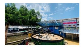
AFWTU system, located at Camp 19, is a multistage treatment process system, containing mechanical, biological, and chemical methods in order to treat the communal wastewater / human waste in the refugee camp. For a normal operation shift of the plant not more than two people are required: A shift leader (skilled) and a second person. The desludging teams are considered separate.
