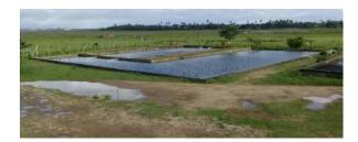
The dumping station is the first module of the Sludge Treatment Site (STS), where the tractors empty the barrel. It is composed of two emptying tanks where the barrel is emptied and its volume measured, with a screen to remove the solid waste, of a channel and of an outlet tank where the scum is trapped.
