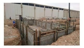
In September 2018 BORDA began construction of a waste water treatment facility in Baharka refugee camp for Iraqi IDP's (Internally Displaced People). The system treats 20 m<sup>3</sup> of grey-water per day. This water comes from the 298 camp dwellings housing 725 families. The treated wastewater replaces the 20 m<sup>3</sup> of fresh water required to irrigate the existing 6 greenhouses inside the camp. The total cost of the project is equivalent to the cost of 3 years of water trucking
