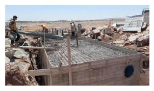
The project piloted a 3-chamber communal septic tank design supported by a study to investigate its efficiency and possible treatment steps that can be added to the system. Implementation was done in partnership with the following implementing partners: ACU, Watan, Saed and Bonyan, with support from different international and funding organizations. The intervention targeted about 14 camps, 4 informal camps and 10 planned camps.
